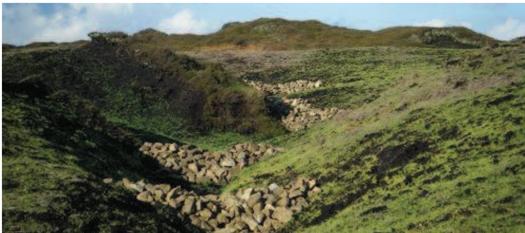
Stone gully blocks and early stage re-vegetation (Derbyshire project)
